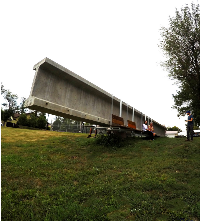
Figure 3. Public Works Beam, the second permanent structure installed through the PCI Grant in Webster, SD. Image credit: DoArch.
